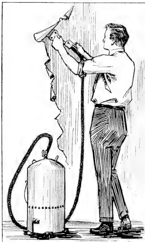
Every bit of wallpaper should be removed before beginning the work of repapering
